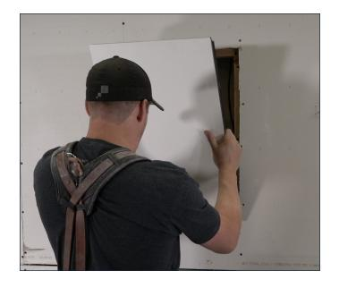
11. Ensure the center of the speaker diaphragm (not the recessed edges) is flush with the surrounding drywall. Adjust shims if necessary.
