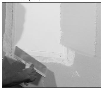
NOTE: DO NOT use fast-setting drywall compound ("hot mud") to cover the speaker; it is not flexible enough to provide a durable finish for invisible speakers. Instead we recommend a lightweight all-purpose joint compound to cover joints and feather up to the surface of the speaker. Lightweight, easy-sand topping compound should be used for covering the speaker.
